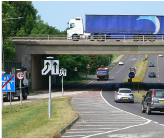
M27 junction 10 and the north going A32, near Fareham. Traffic on the A32 has been moved to the outer lane to provide a protected entry lane for merging traffic.
