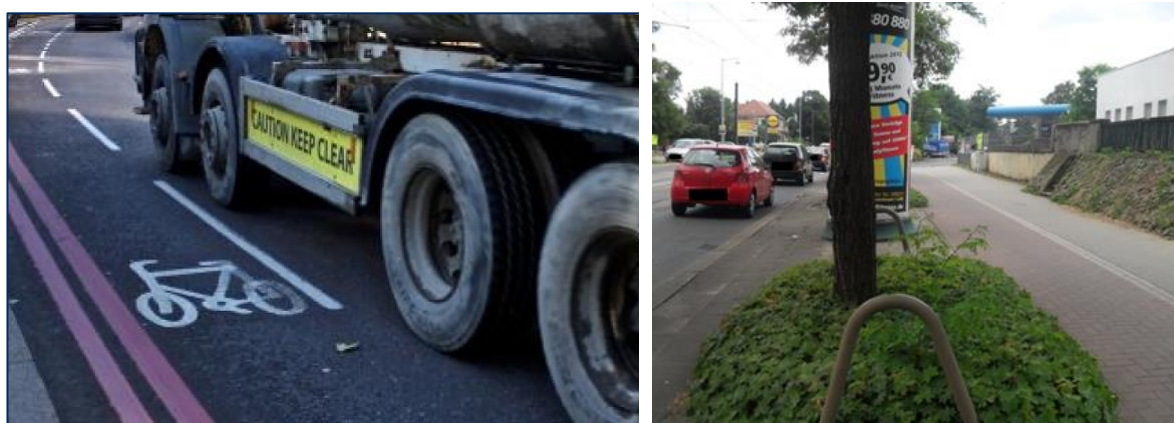
Figure 8-2: Examples of separated cycle lanes with potential line of sight obstruction in Germany. Source London on left (Knight, 2017) & Berlin on right (Schreck & Seiniger, 2014).
