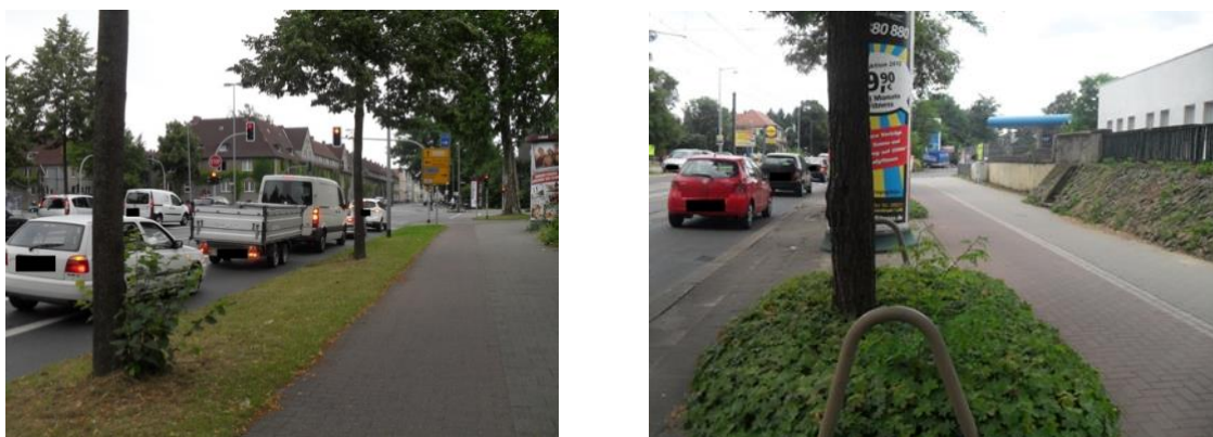
Figure 4-5: Examples of separated cycle lanes in Germany. Source (Schreck & Seiniger, 2014)
